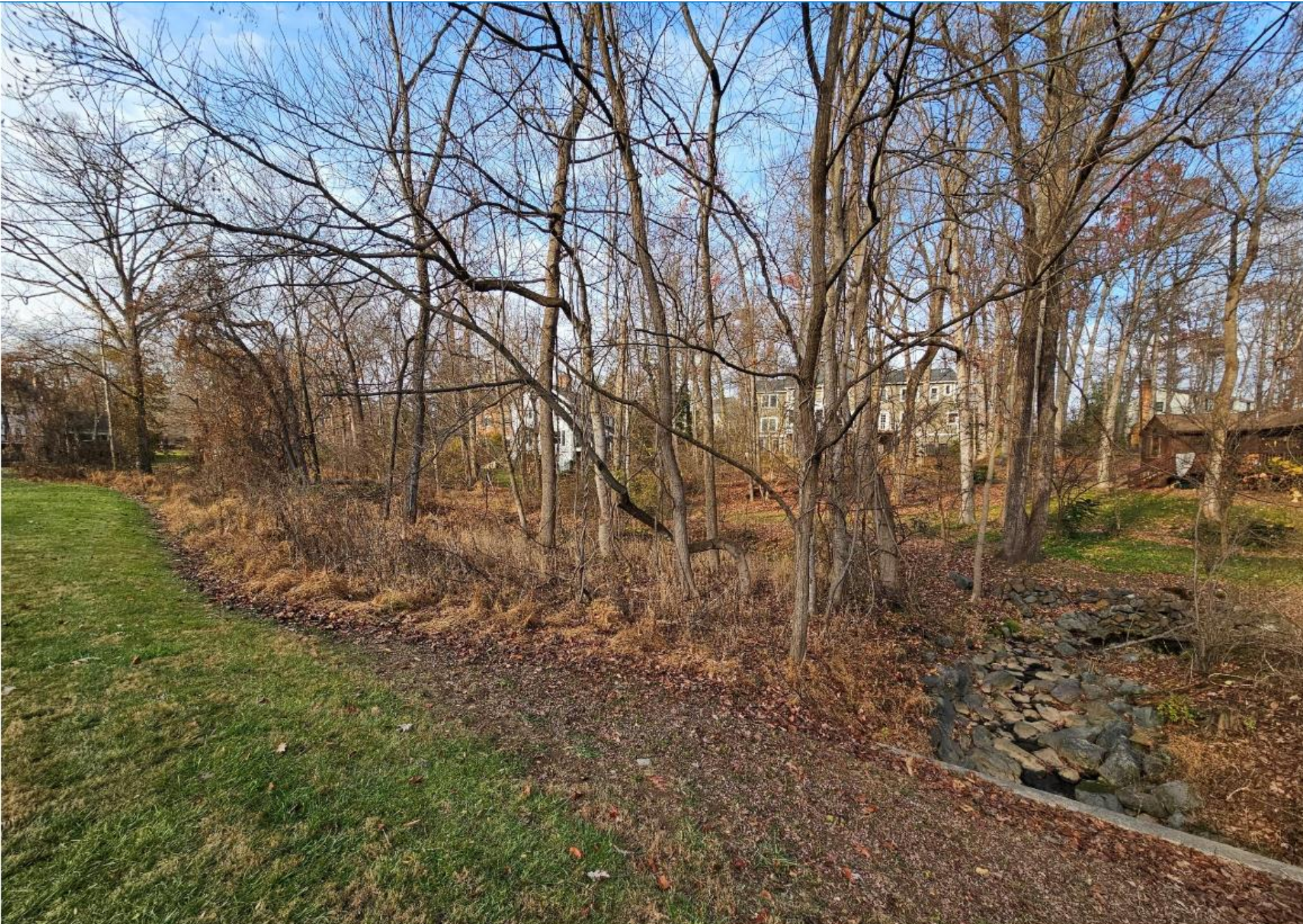
Picture #3 – Pond Outfall Along Northern Embankment
