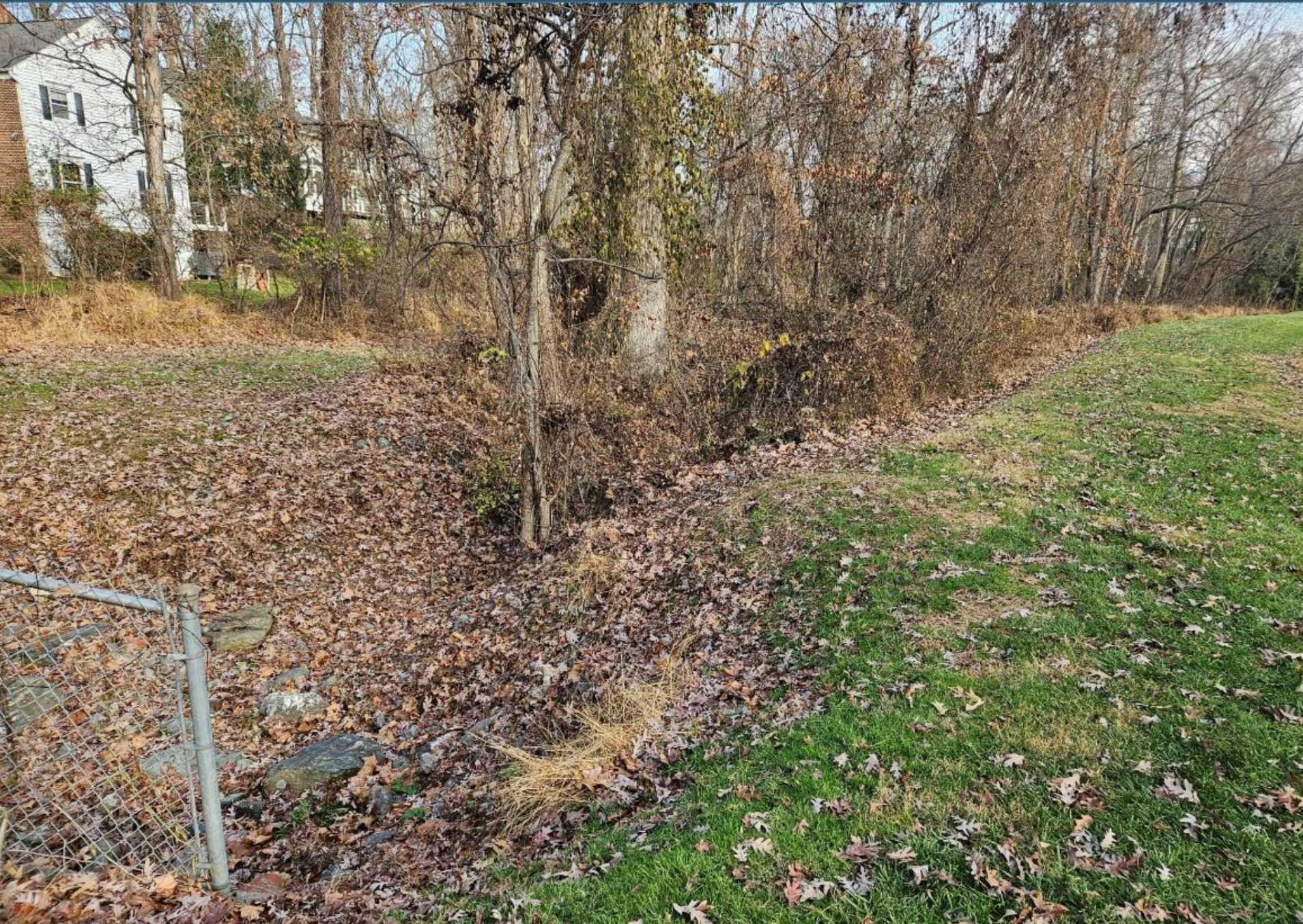
Picture #1 – Side Channel End Wall Along Northern Embankment
